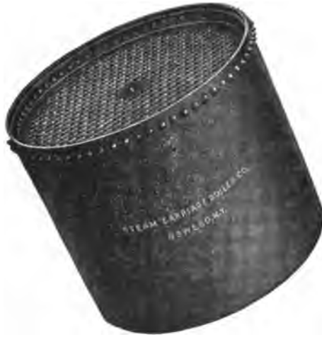
FIG. 146.—Bottom View of a Type of Boiler shown in Fig. 145, exhibiting the method of riveting in the lower tube plate.
